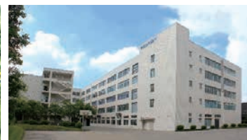
R&D Center in Guangzhou
